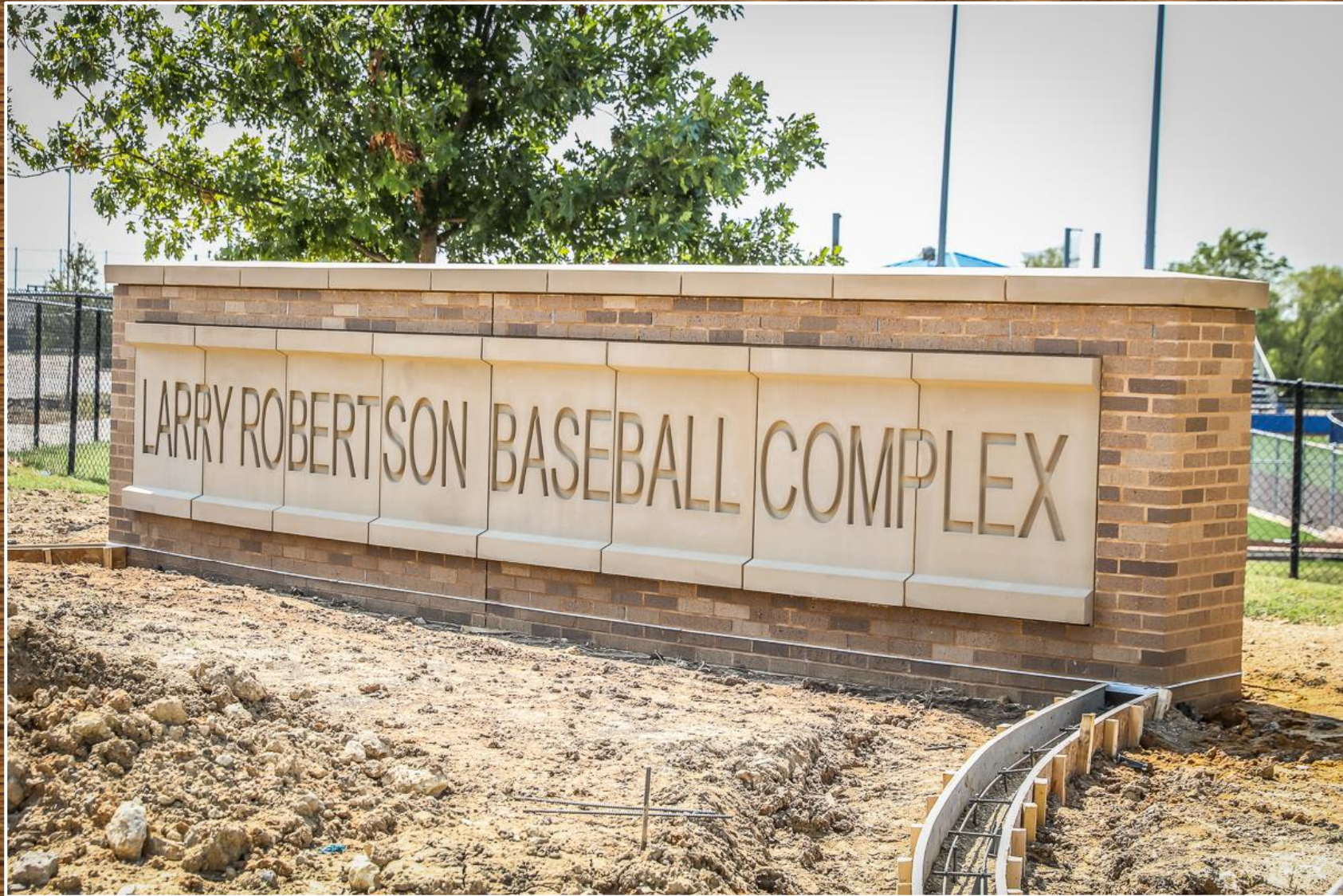
Work continues on the monument sign.
